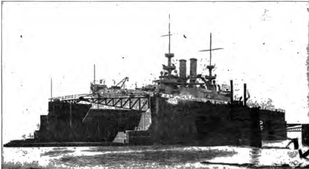
FLOATING DOCK SHOWING BATTLESHIP ILLINOIS IN PLACE. This dock was built by the Government for use at New Orleans.
